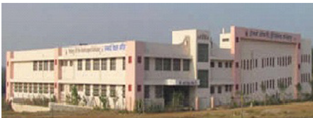
The school building of HoH
